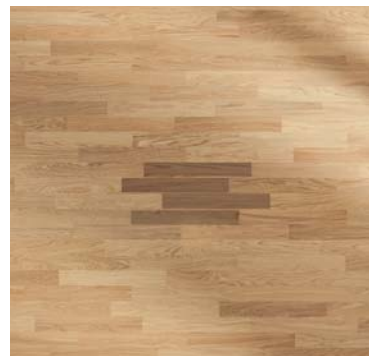
Regular pattern (English bond) Here, the strips are installed in parallel rows, which are offset by half a strip length.
