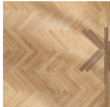
Border Inlay Traditional installation pattern that was widespread in upper-class residences in the 19th century.
